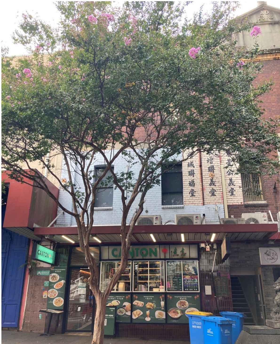
Figure 26. View of 50 Dixon Street. Source: HAA, 2024.
