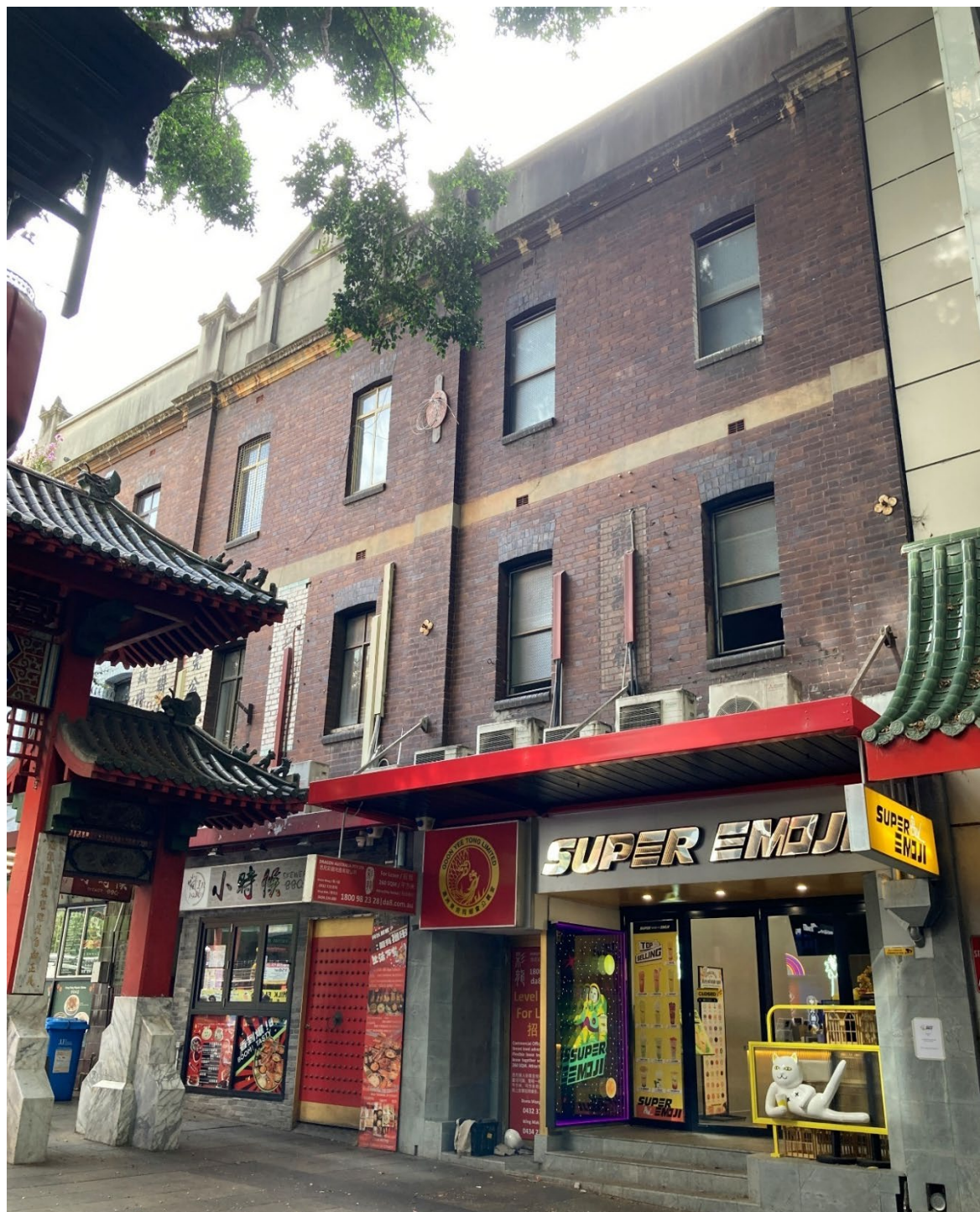
Figure 24. External view of 50-54 Dixon Street. Source: HAA, 2024.
