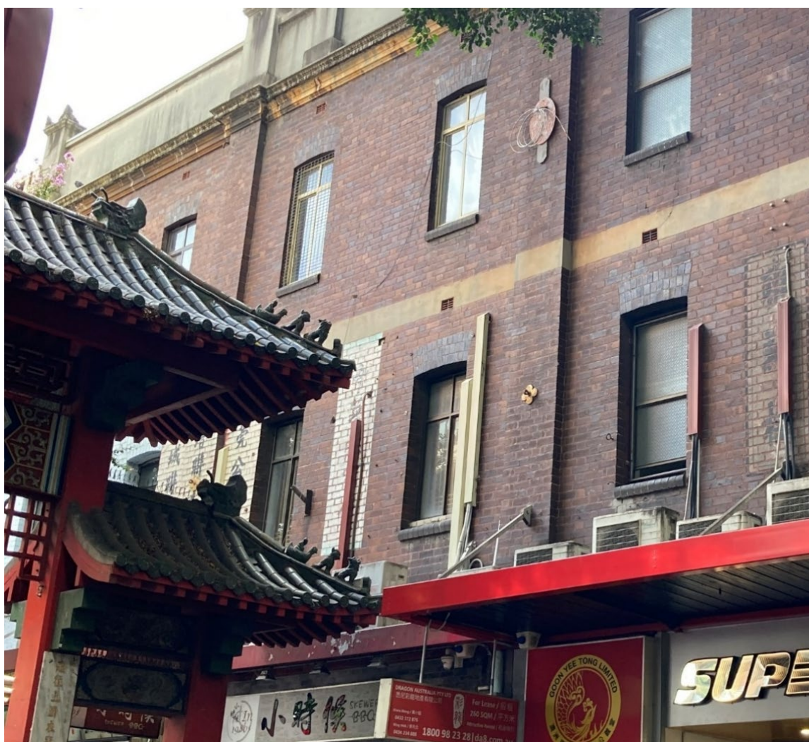
Figure 29. View of 52 Dixon Street. Source: HAA, 2024.
