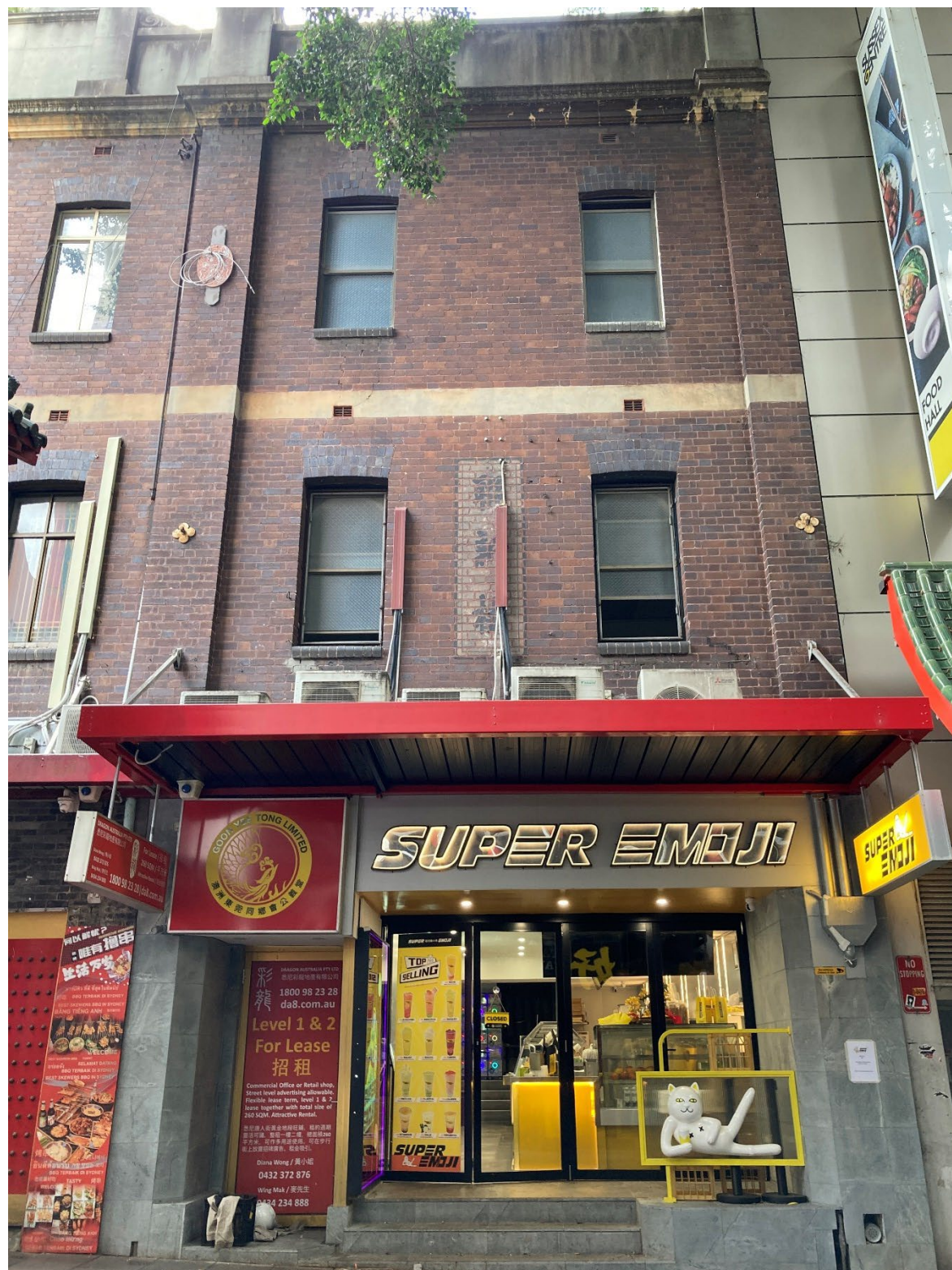
Figure 30. View of 54 Dixon Street. Source: HAA, 2024.
